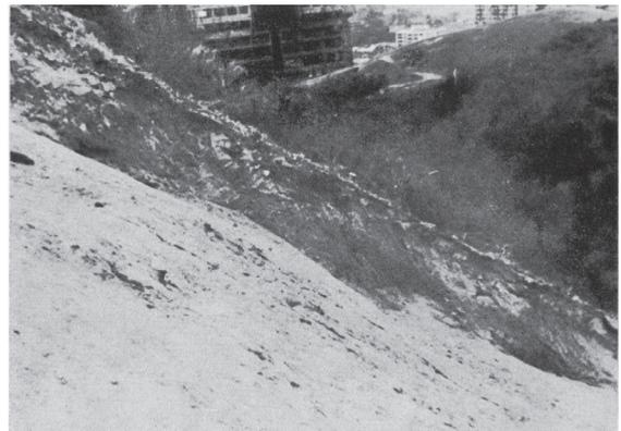
Figure 4. View showing the shallow depth of the slide and layers parallel to the slope
